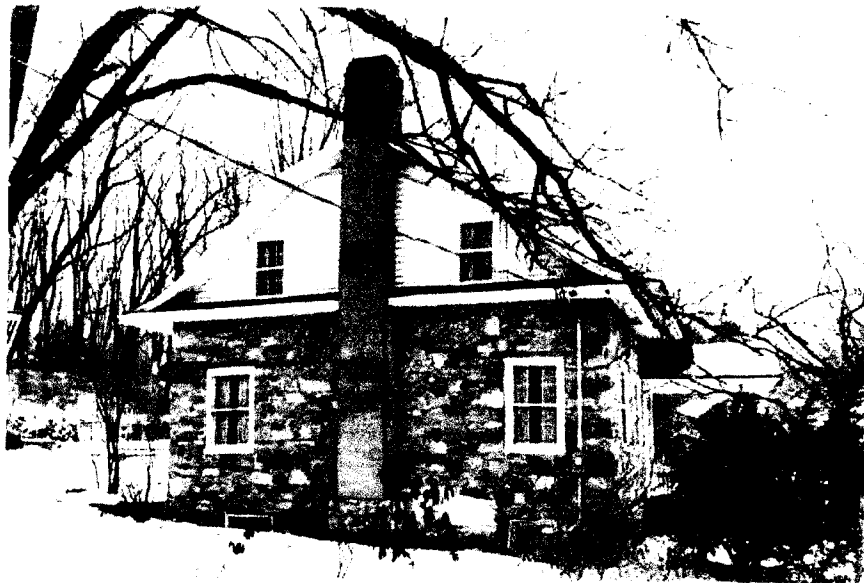
Photograph 2 West Elevation Original increment showing Page alterations to gable end and modern concrete chimney.
