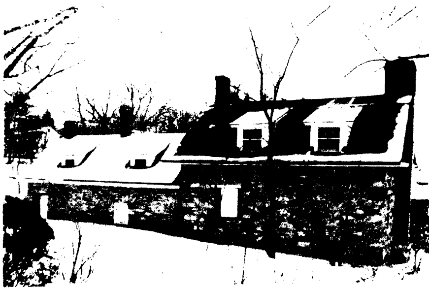
Photograph 4 North Elevation Original increment, first and second additions REAR
